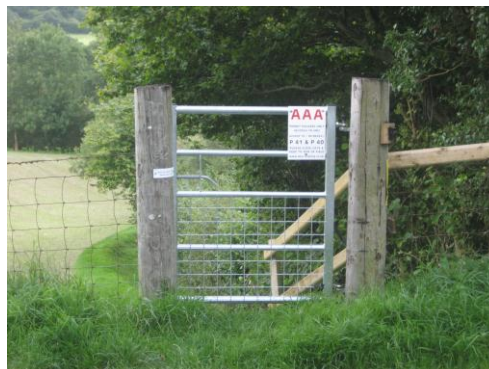
One of the new gates (this one at Mill Pool)
