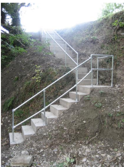
The new steps at Irmhytage
